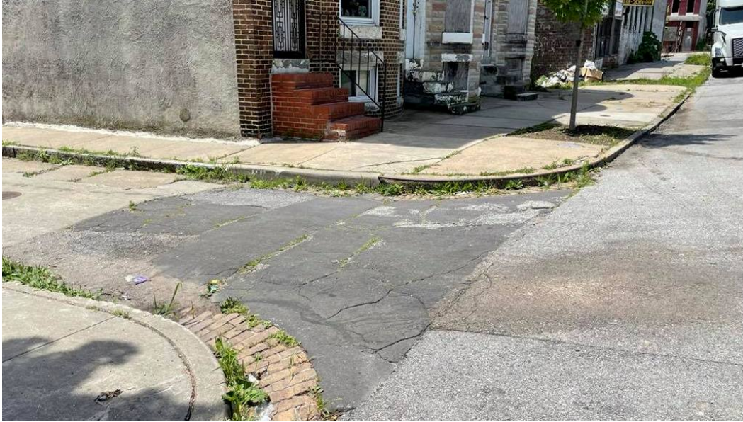
Curb ramp were never installed at the Bruce Street intersection with Westwood Avenue in West Baltimore. (Fern Shen)
