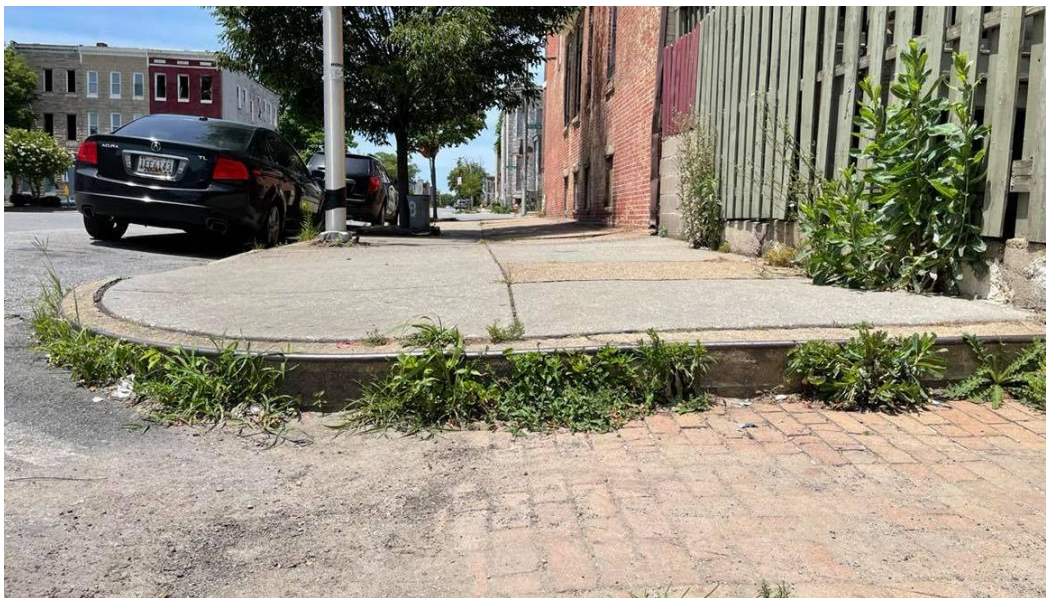
No curb ramp at all at this spot on Westwood Avenue in West Baltimore. (Fern Shen)
