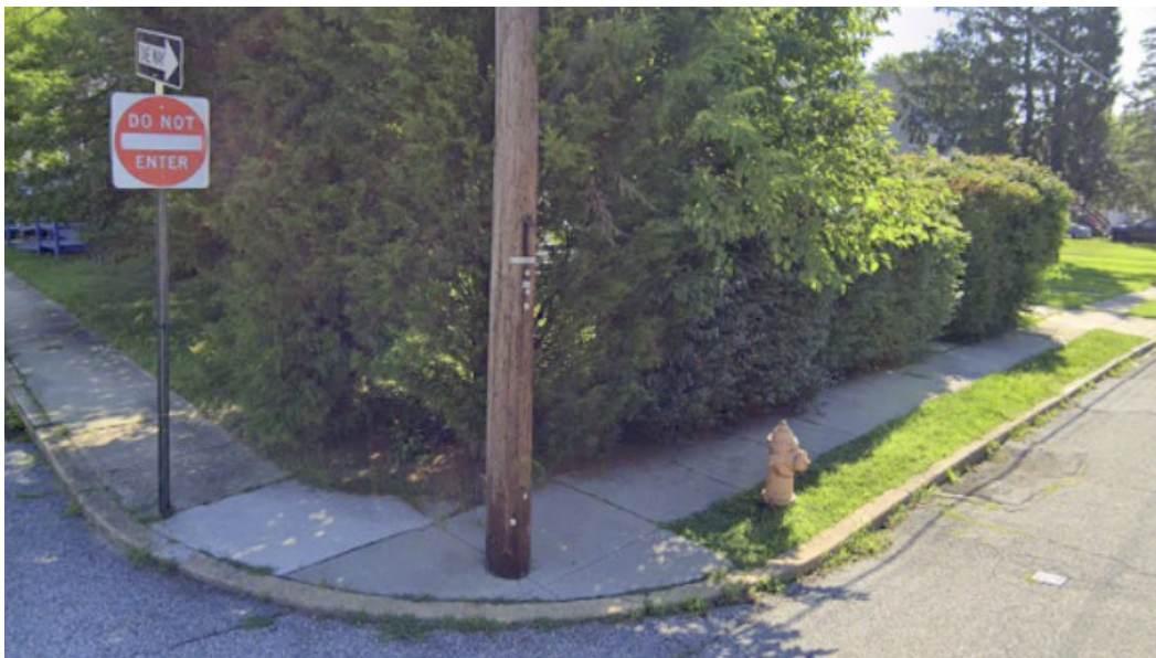
No curb ramp – and a telephone pole blocking the sidewalk – make this spot in northeast Baltimore especially non-ADA-compliant. (Google/dralegal.org)
